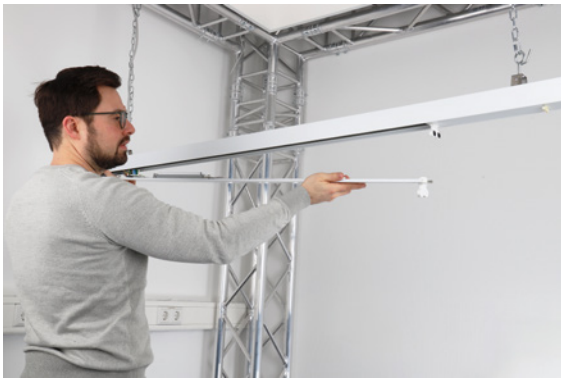
1 - old light inserts removed [wiring remains in]
